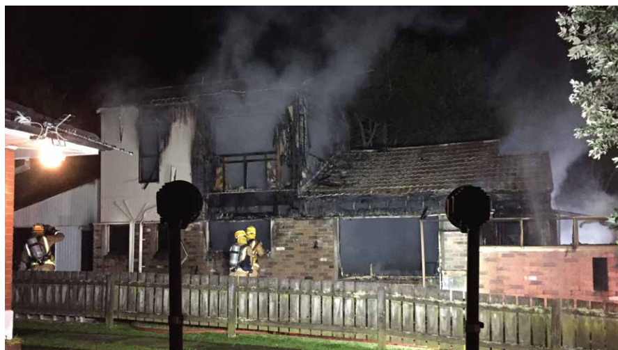
House Fire - Lighting
